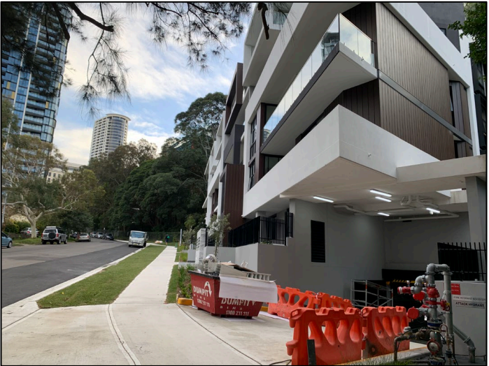
Figure 8 – Flat Building Along Duntroon Ave Looking North Source: Mecone
